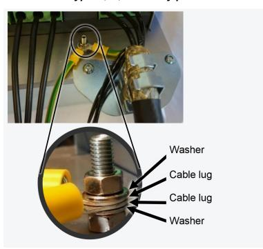
Connect the protective earth from the motor and the mains together on the earth terminal using cable lugs.
